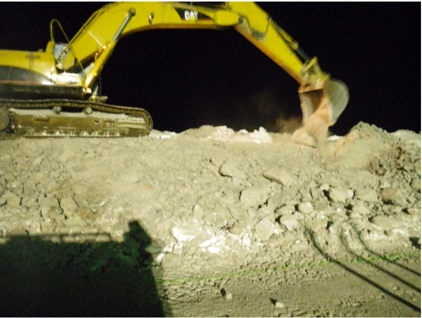
Photo 12: CAT 330 excavator placing ROQ material on downstream side of the dam.
