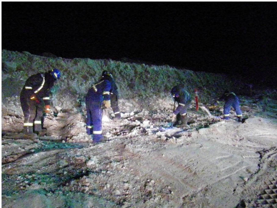
Photo 7: Labourers shoveling 5/8" core material from the HDPE liner on the upstream side.
