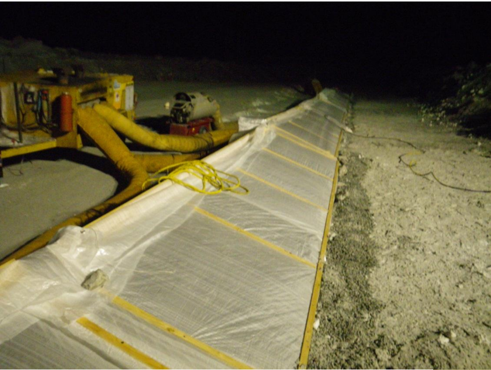
Photo 8 (Left): Looking at Herman Nelson heaters and hotbox heating liner hinge area. Photo looking north east along trench.
