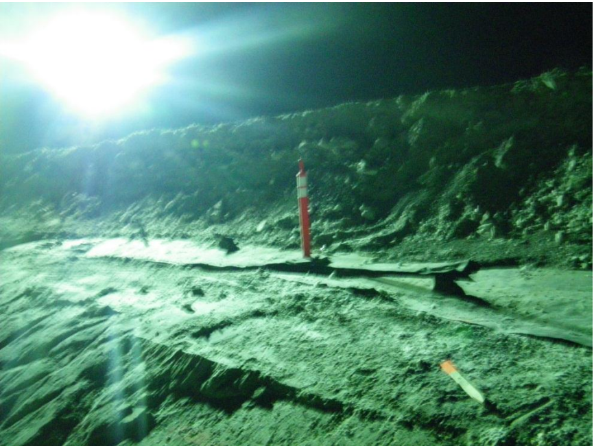
Photo 11: A closer look at the exposed HDPE.
