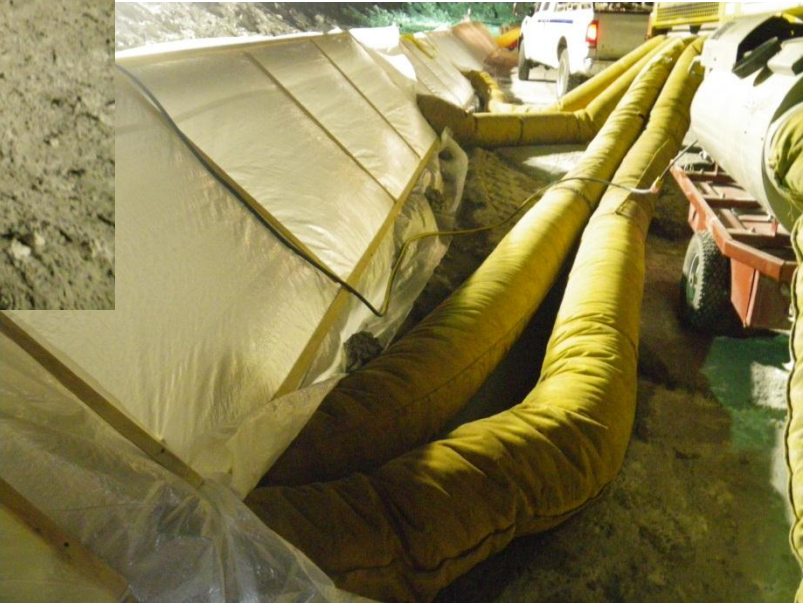
Photo 9 (Below): Some melting of the core material was observed where the trunks for the heaters rested on the ground. Rocks were used to bring the trunks off the ground.
